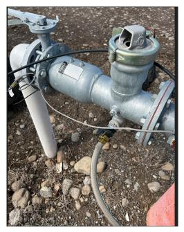
Examples of a backflow prevention devices using check valve, vacuum relief and low-pressure drain.
