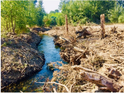
The Walla Walla Basin Watershed Council's Lamson Habitat Side Channel Entrance Construction Project converted a dry side channel to perennial flow.
