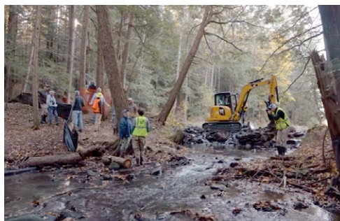
Sucker Brook Restoration by the Massachusetts Division of Ecological Restoration . Still from video .
