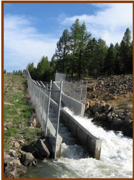
Photo 3. Bates Pond fish ladder. Courtesy of ODFW.
