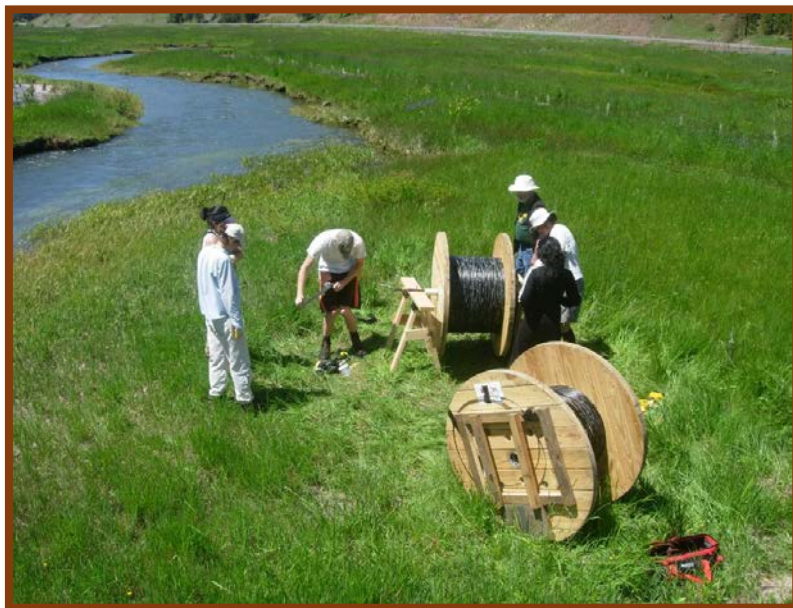
Photo 13. Wiring monitoring equipment. Courtesy of CTWSRO.
