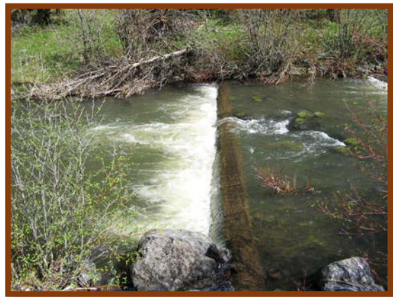
Photo 7. Log weir in Camp Creek. Courtesy of ODFW.
