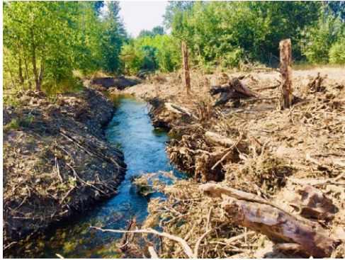
The Walla Walla Basin Watershed Council's Lamson Habitat Side Channel Entrance Construction Project converted a dry side channel to perennial flow.
