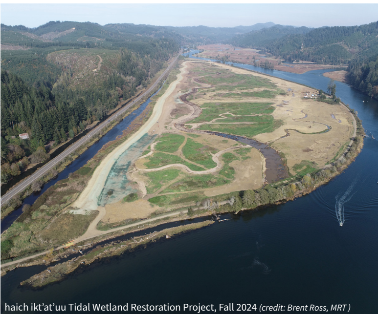
haich ikt'at'uu Tidal Wetland Restoration Project, Fall 2024 (credit: Brent Ross, MRT)
