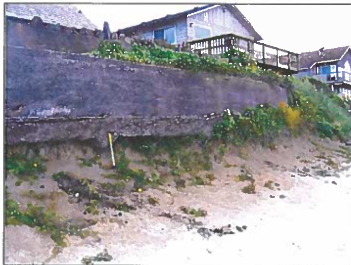
Photo 3: Undated photo of site beachfront and former seawall, presented in Witter et al (2009) as an “example of a seawall in Cannon Beach that has been undermined by wave erosion”.
