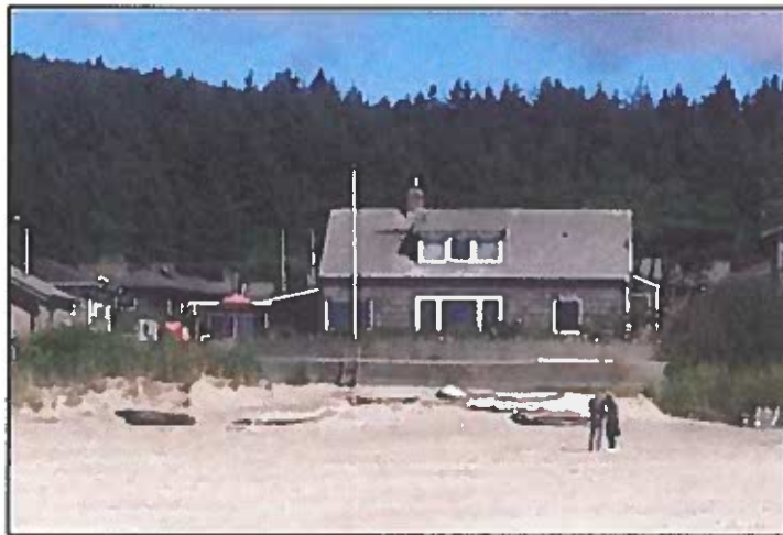
Photo 2: Undated historical photo provided by the property owner, looking east at the subject property and seawall (note that the beach elevation at the time of the photo is substantially higher than the current beach elevation.)
