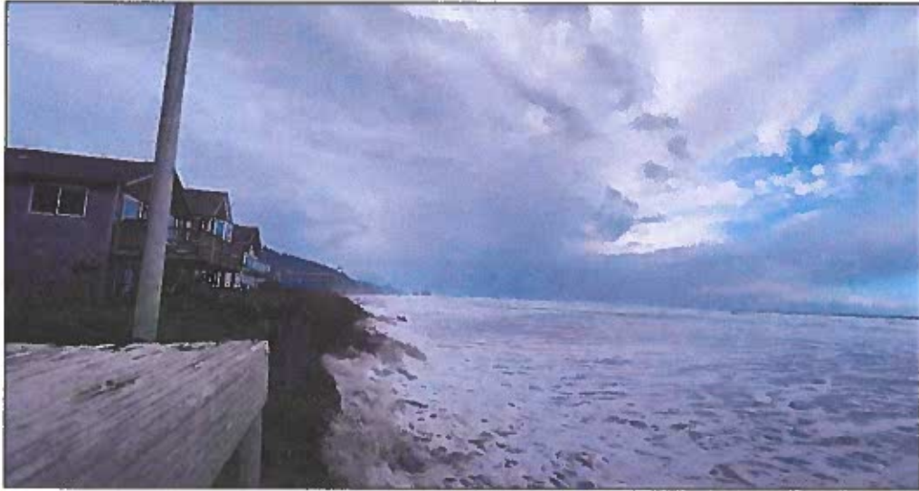
Photo 4: Photos of site beachfront in January 2022 showing ocean runup at high tide, facing north (provided by Stephen Day, property owner).
