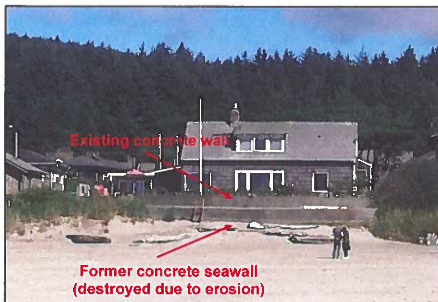
Photo 3: Undated historical photo provided by the property owner, looking east at the subject property and seawall (note that that the beach elevation at the time of the photo is substantially higher than the current beach elevation.)
