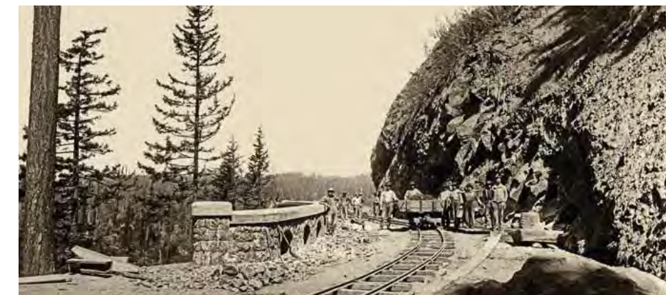
Historic Columbia River Highway Construction
