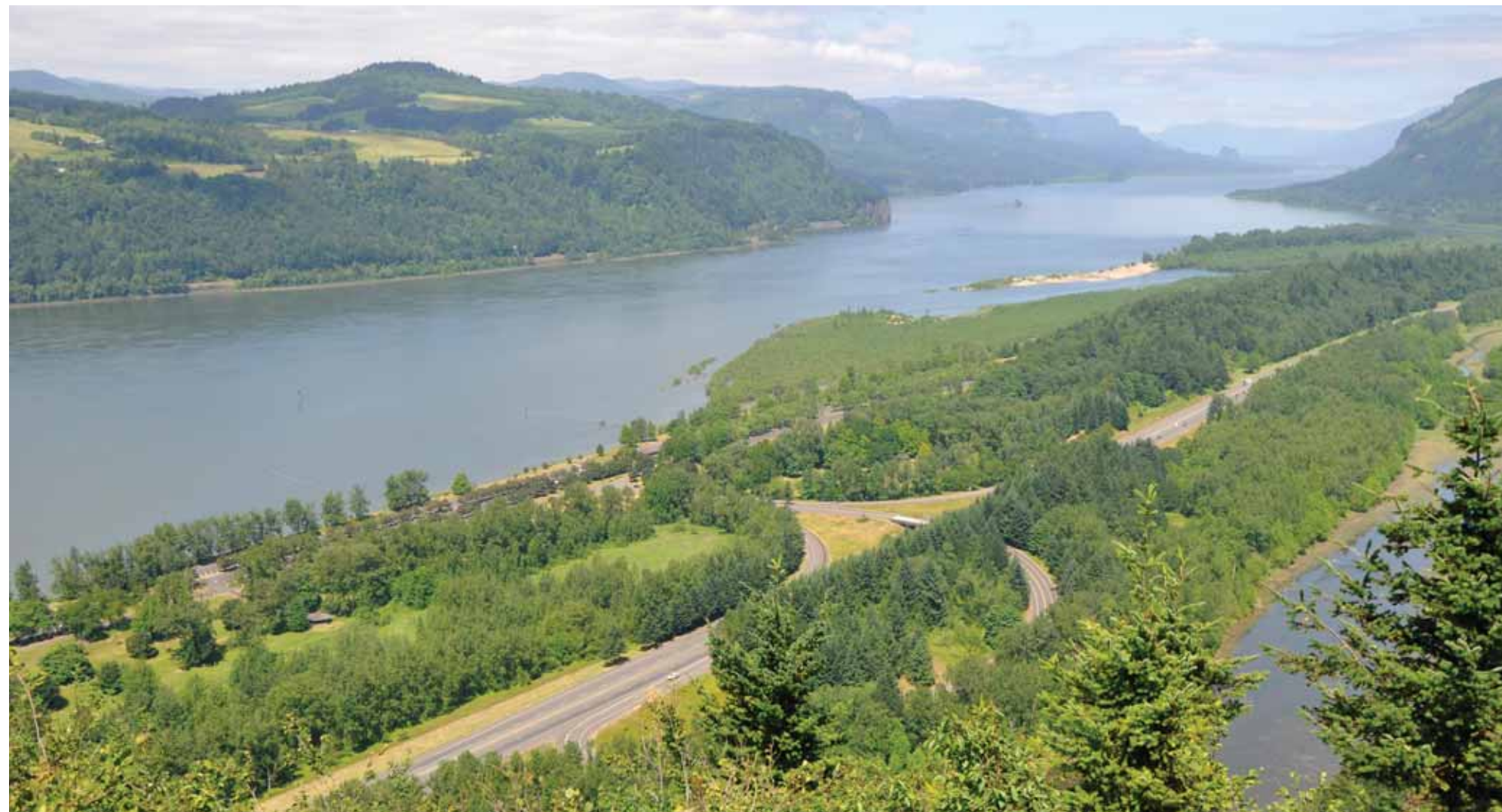
Rooster Rock's Beach Was Severely Eroded During Flooding in 1996 (Image from Crown Point)
