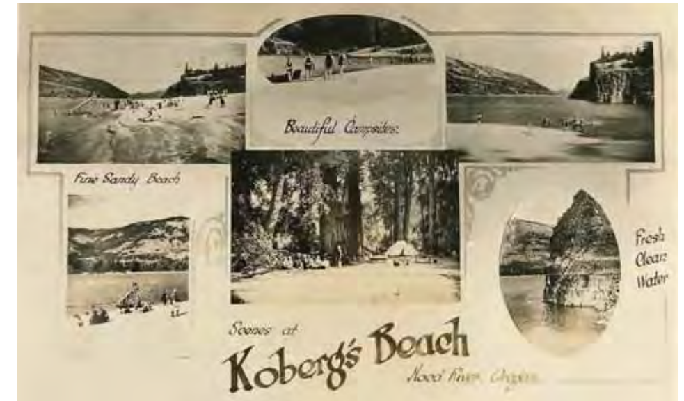
An Advertisement for Koberg Beach, Prior to the Construction of Bonneville Dam
