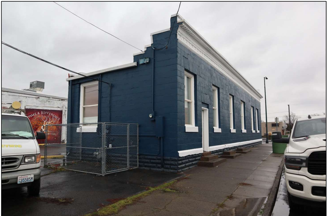
Photo 2 of 19. West and south elevations, camera facing northeast.
