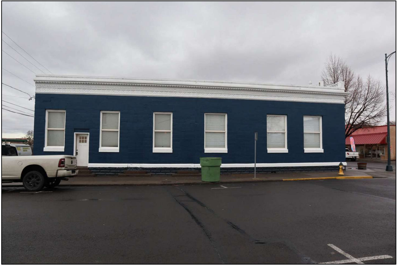
Photo 7 of 19. South elevation, camera facing north.
