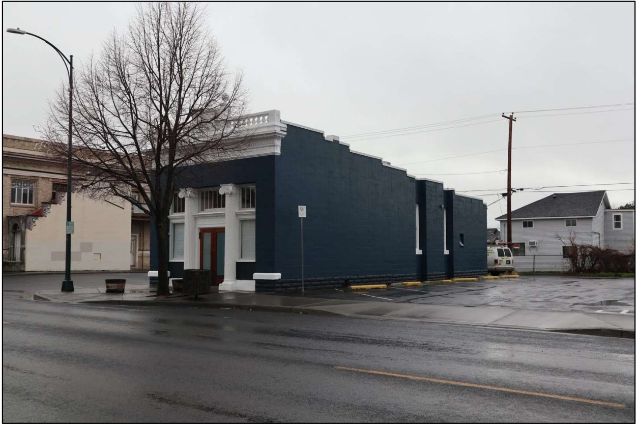
Photo 1 of 19. East façade and north elevation, camera facing southwest.
