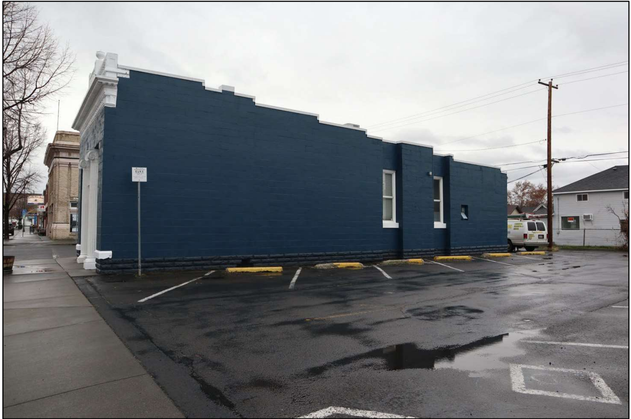
Photo 5 of 19. North elevation, camera facing south.
