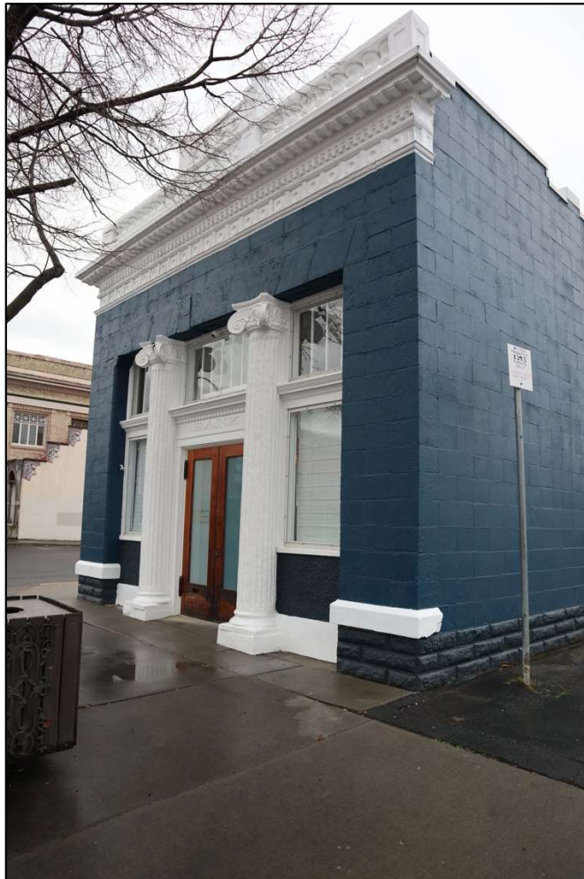
Photo 12 of 19. East façade, camera facing southwest.
