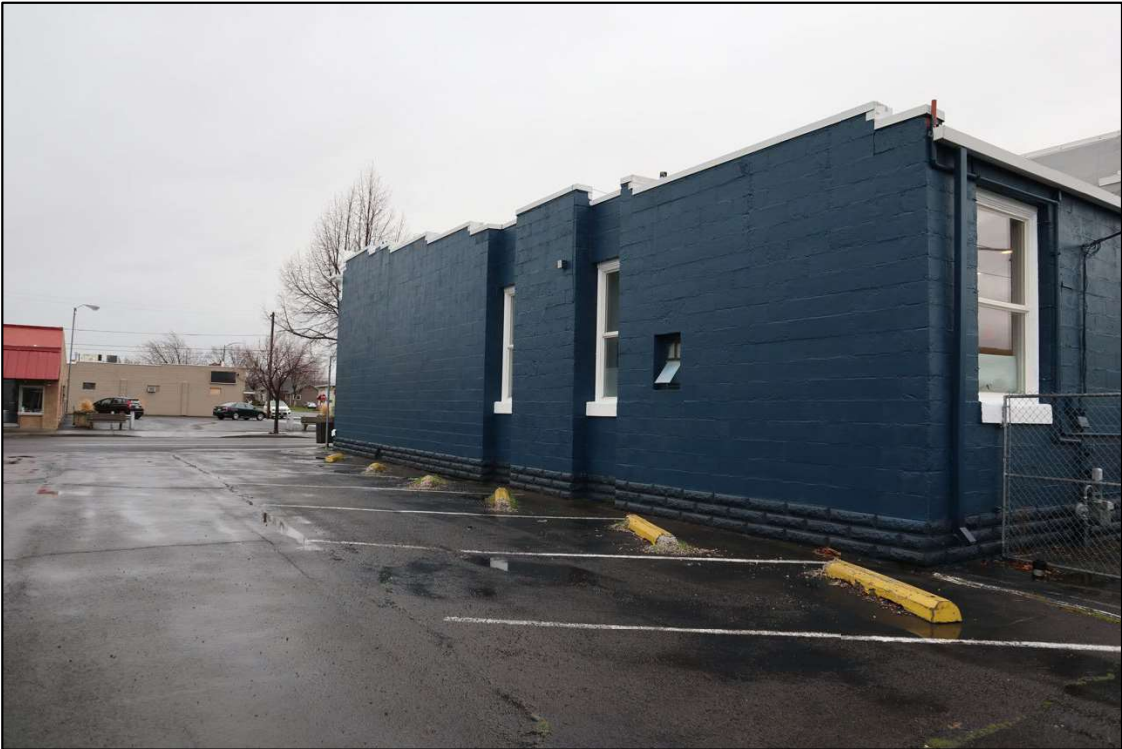
Photo 4 of 19. North elevation, camera facing southeast.
