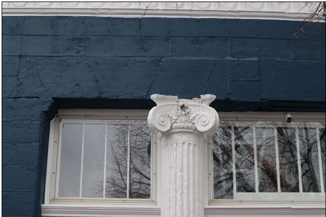
Photo 10 of 19. Column detail, camera facing west.
