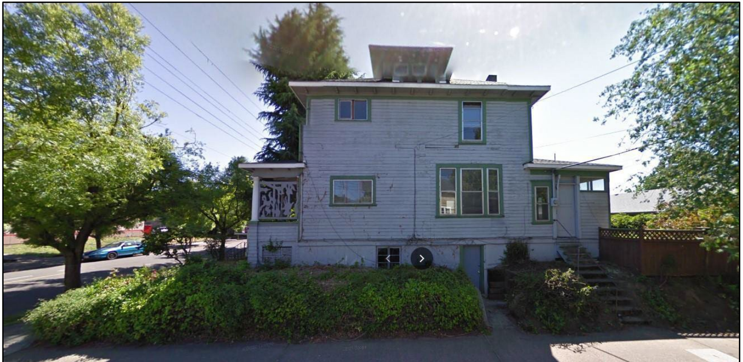
Figure 18. 2009 photograph of Juniper House, prior to 2010 renovations. Photo from SE 20 th Ave facing east, view of the west façade. Note the ghost shadows around the three-windows showing the original location of the oriel window. Note the rear porch door location and fixed windows on the corner that were removed in 2010. Source: Google Streetview.
