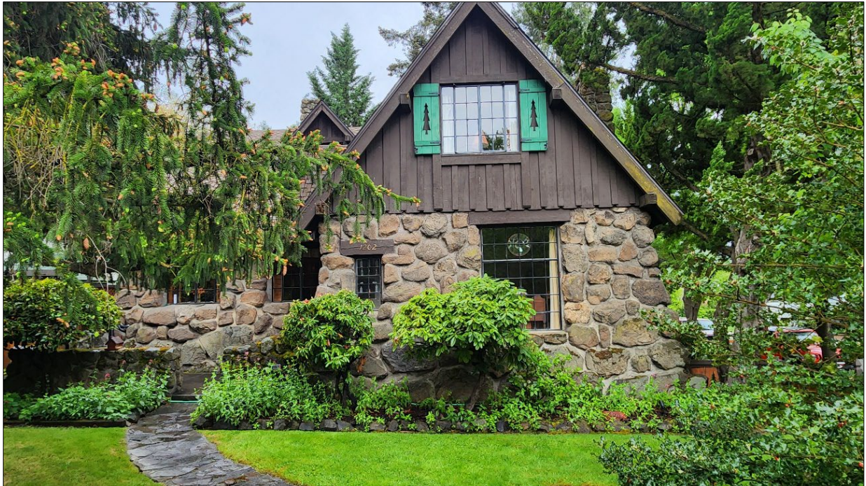
Photograph 3 of 12: OR_JacksonCounty_Lee-JanouchHouse_0003 North elevation, looking south, from entry walkway (May 2024).
