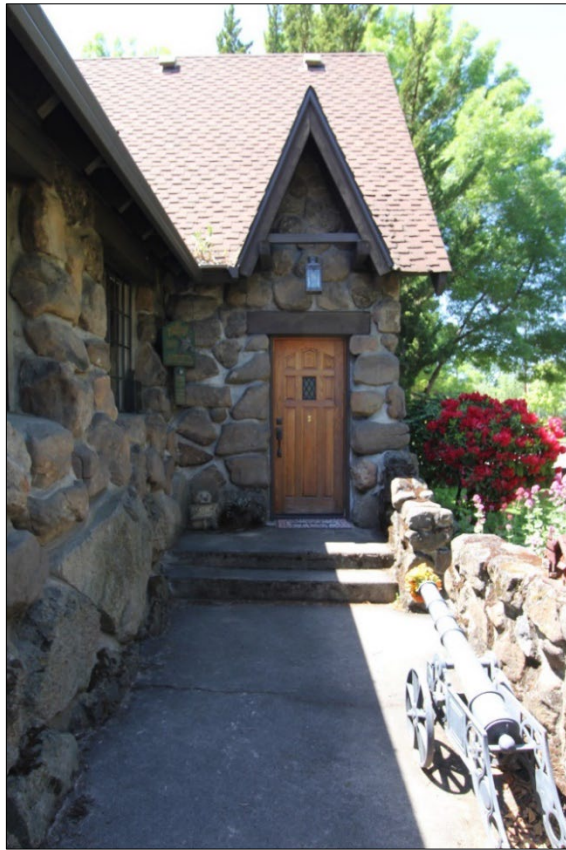
Photograph 9 of 12: OR_JacksonCounty_Lee-JanouchHouse_0009 Main Entry, looking west (May 2024).
