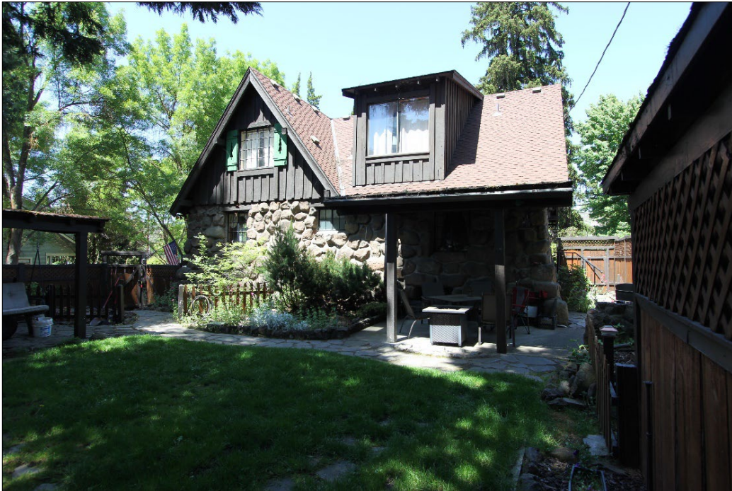
Photograph 5 of 12: OR_JacksonCounty_Lee-JanouchHouse_0005 South (rear) elevation, looking northwest from rear property line (May 2024).
