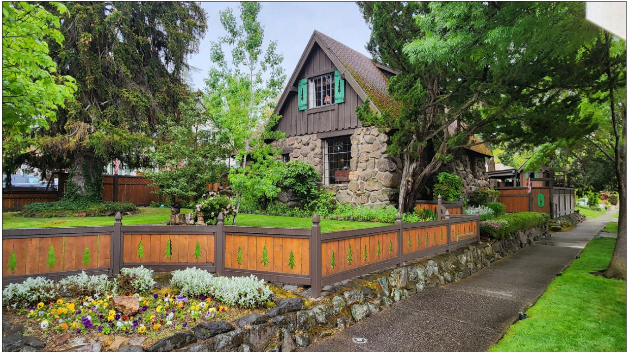
Photograph 1 of 12: OR_JacksonCounty_Lee-JanouchHouse_0001 Looking southeast from corner of Willamette Avenue and East Main Street (May 2024).
