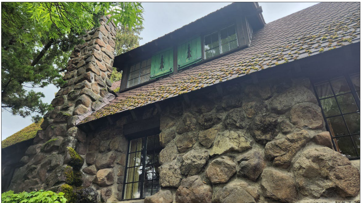
Photograph 8 of 12: OR_JacksonCounty_Lee-JanouchHouse_0008 West elevation, Chimney and dormer detail (May 2024).
