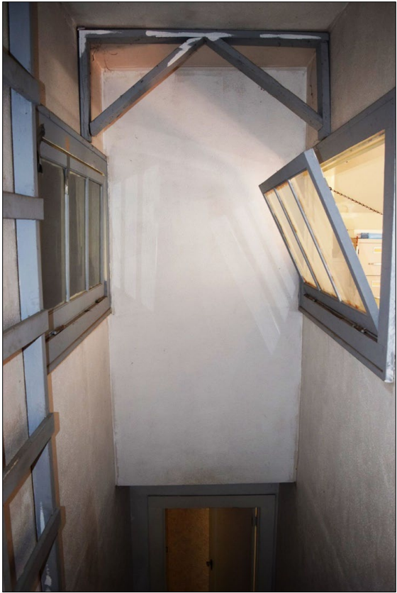
Photo 15 of 15: OR_ClackamasCounty_McLeanHouse_0015 Interior, at top of attic stair looking southeast.
