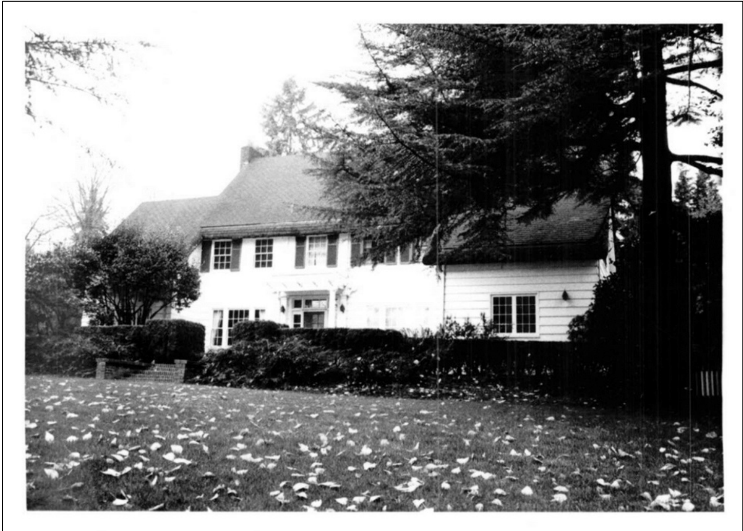
Figure 13: 1984 architectural survey image, "McLean Residence," Cultural Resource Survey Form by Pinger/Altier team.
