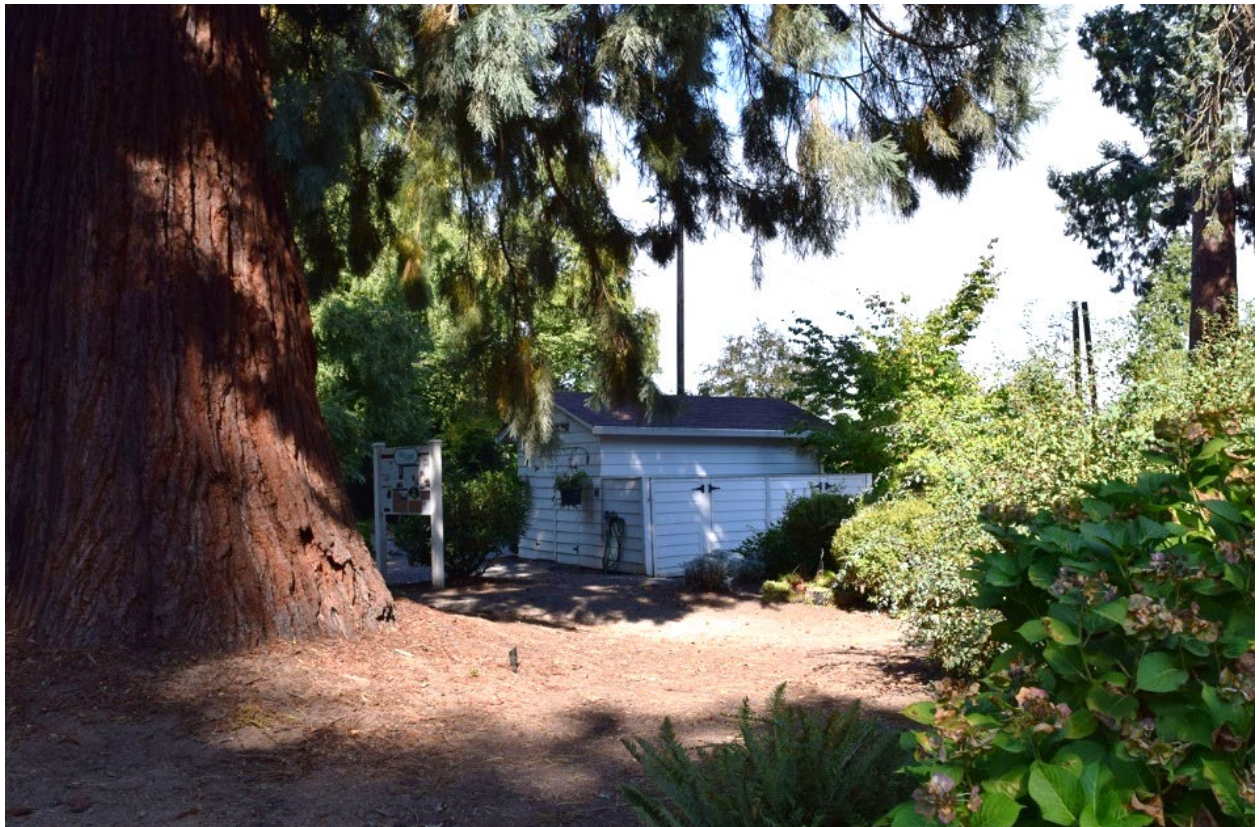
Photograph 6 of 15: OR_ClackamasCounty_McLean,Dr.EdwardandAnne,House_0006 Looking north/northeast at shed; parking lot beyond is not visible.
