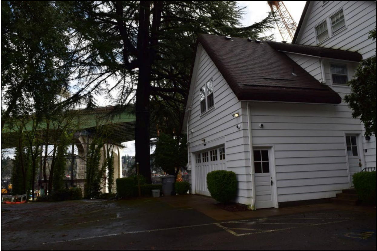
Photograph 3 of 15: OR_ClackamasCounty_McLean,Dr.EdwardandAnne,House_0003 Looking south at garage and kitchen doors.
