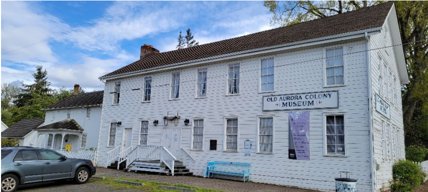
2022 Ox Barn with CeDUR composite roofing material
