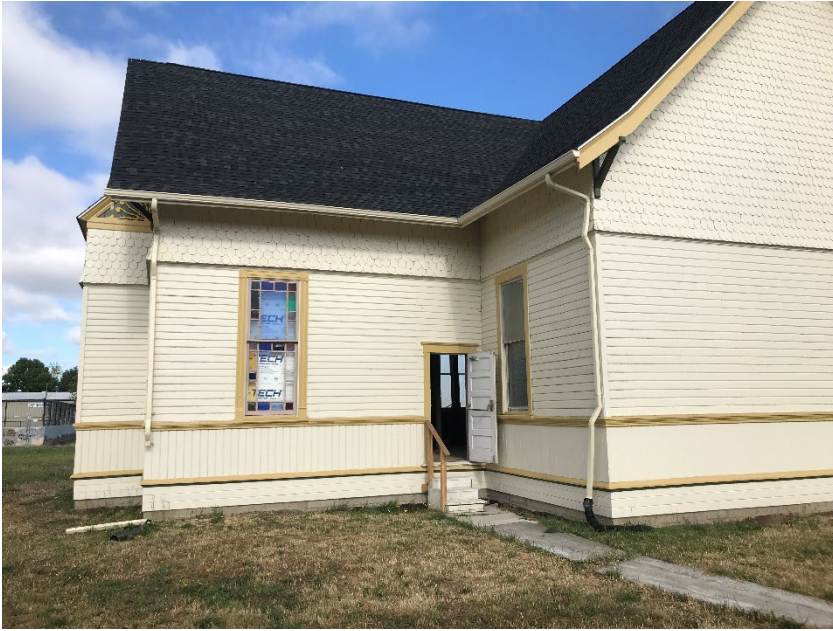
Southeast Façade Showing Subject Window
