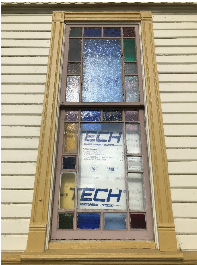
Subject Window – Exterior View
