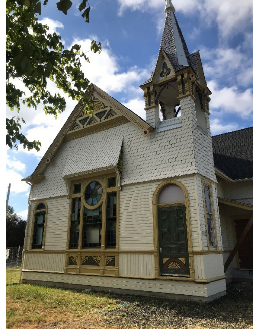
North Façade Showing Restored Windows
