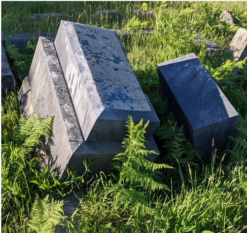
William & Rebecca Craig (B87-15): representative gravestone in need of leveling and resetting in mortar
