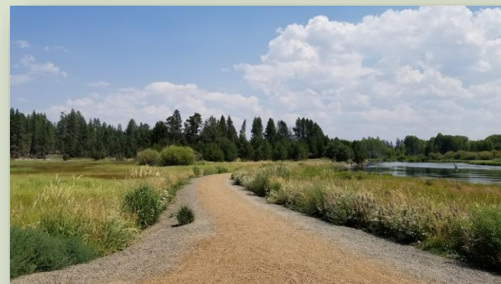
Deschutes National Forest, Ryan Ranch Accessibility Upgrades
