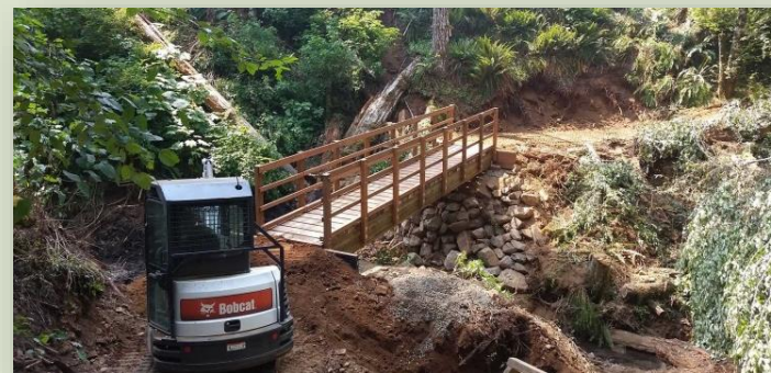
Oregon Department of Forestry, Tillamook State Forest Bridge Replacements
