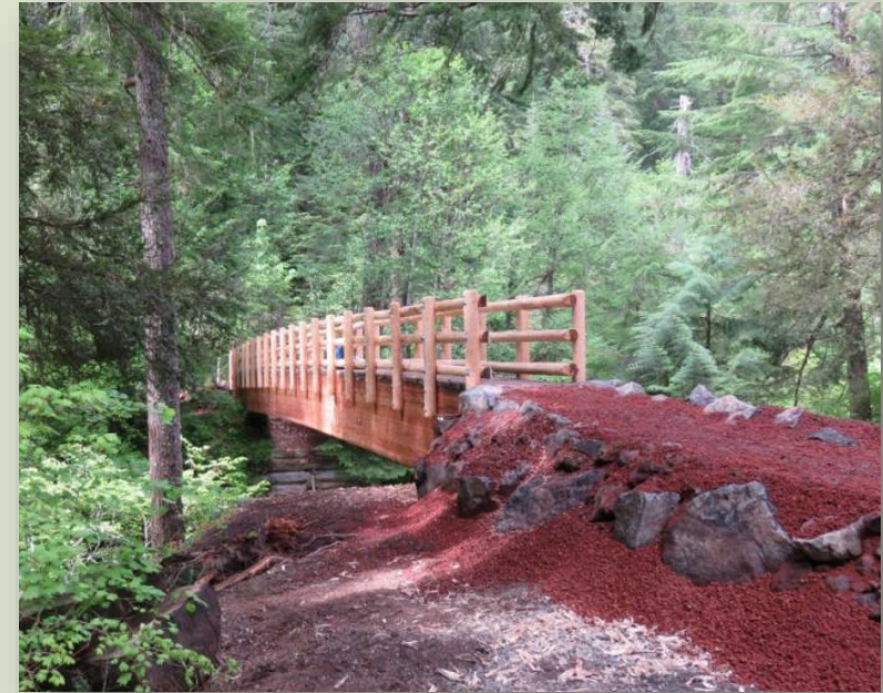
Willamette National Forest, McKenzie River Trail Bridge Replacements
