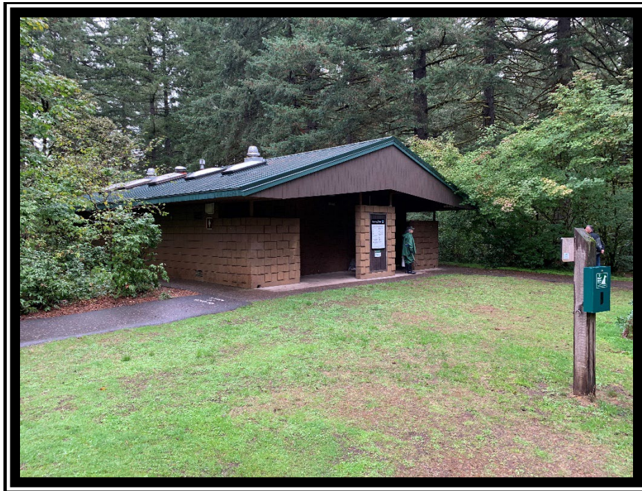
Figure 1 – Existing restroom building.
