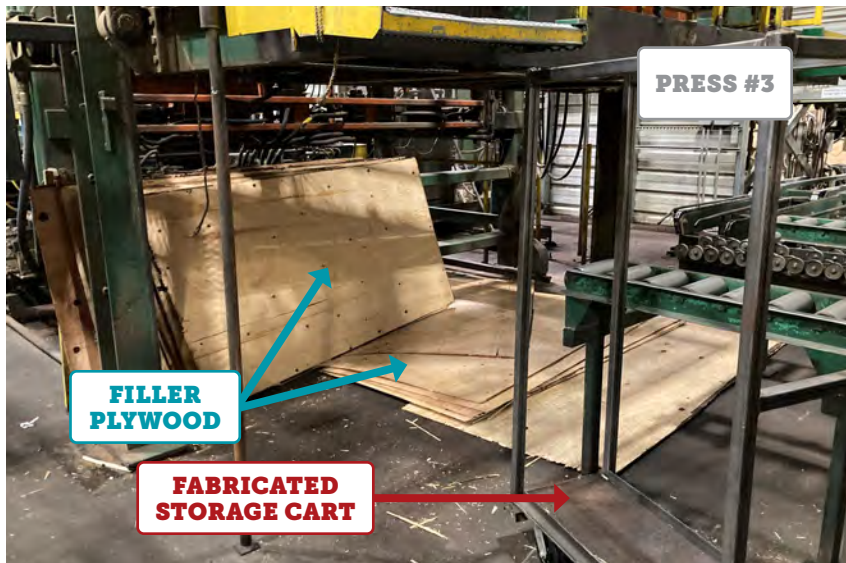
There were 26 pieces of rough-cut filler plywood - 100 inches by 50 inches - stored on the cart when the incident happened. The combined weight of the cart and the filler plywood was 1,117 pounds.
