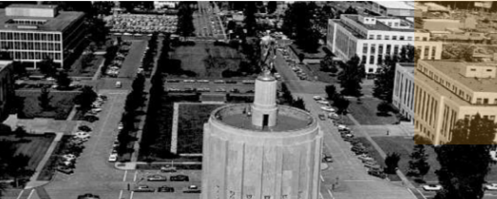
This aerial photo, taken in 1972, shows Oregon's Capitol.
