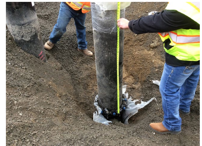
The riser resting in the gland. Note that the blue hex heads are still intact.
