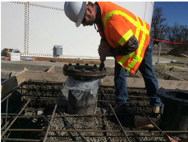
The position of the victim when the riser thrust upward and struck him in the chest.
