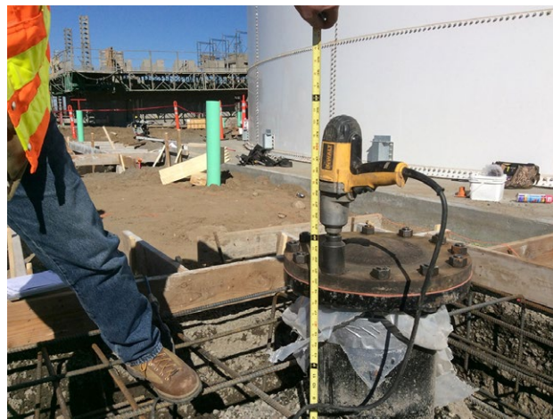
The electric-powered impact driver on one of the bolts.
