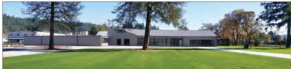
The newly remodeled Oregon Military Mussem at Camp Withycombe in Clackamas Oregon.
