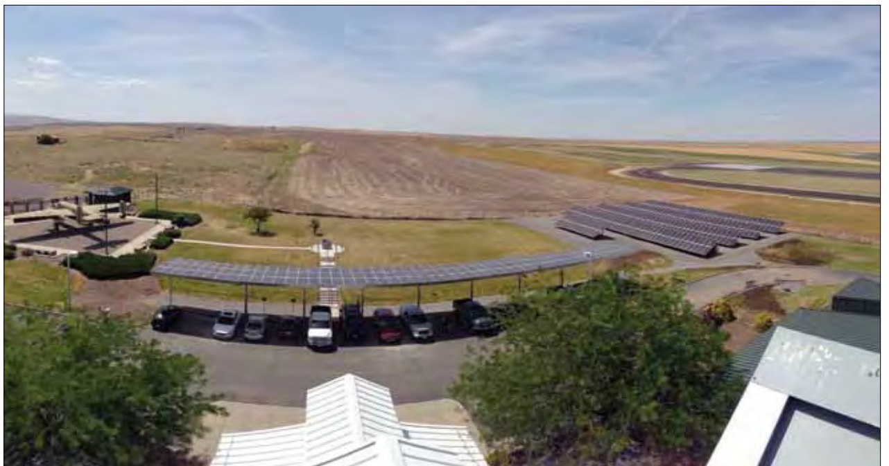
A solar photovoltaic (PV) array was recently installed at the Army Aviation Support Facility (AASF) in Pendleton, Oregon. The 150-kilowatt solar system provides renewable electricity for the helicopter hangar utilizing 475 Oregon-made solar panels divided between a ground mounted system and a carport structure that also provides weather protection for parked vehicles.
