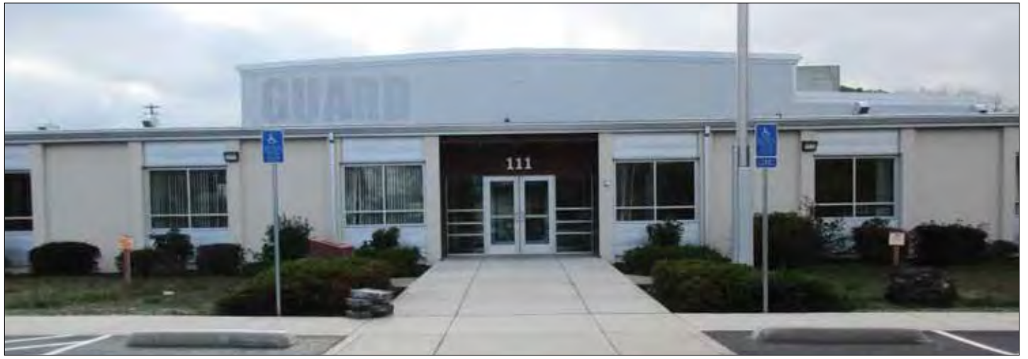
The newly renovated Roseburg Armory is more modern, earthquake safe and energy efficient. This project is one of many energy conservation and renewable energy projects that are being implemented at Oregon Military Department facilities across the state as part of the U.S. Army Net Zero Energy effort to be more energy efficient and energy secure.
