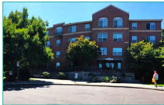
New Addition North Building Constructed in 2000
