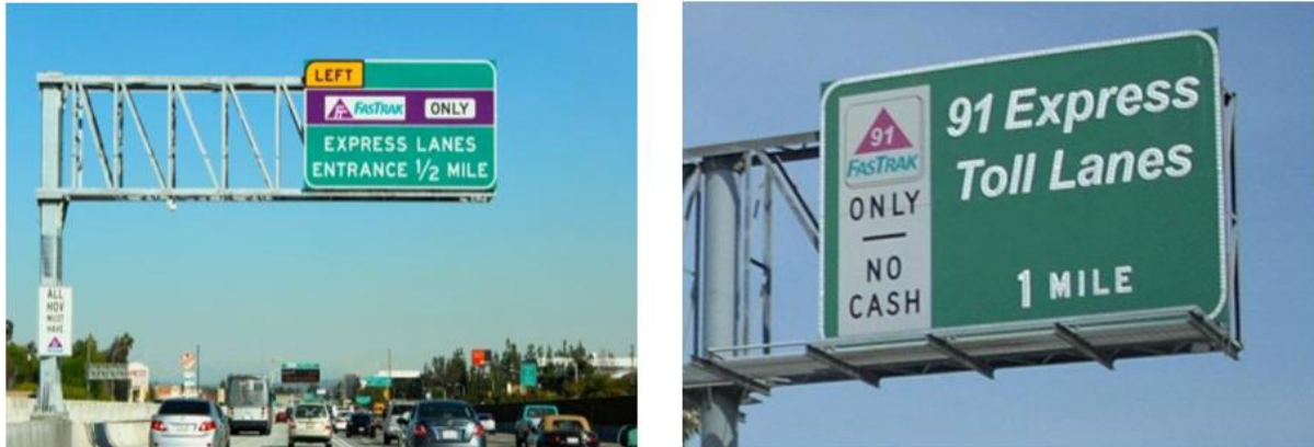
Figure 12: Express Lane Entrance Signage
