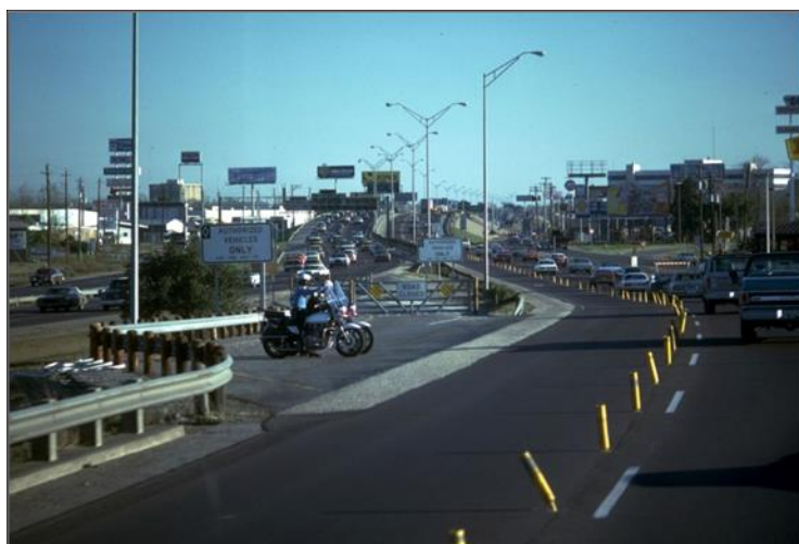
Figure 9: I-45 Enforcement Area in Houston, TX
