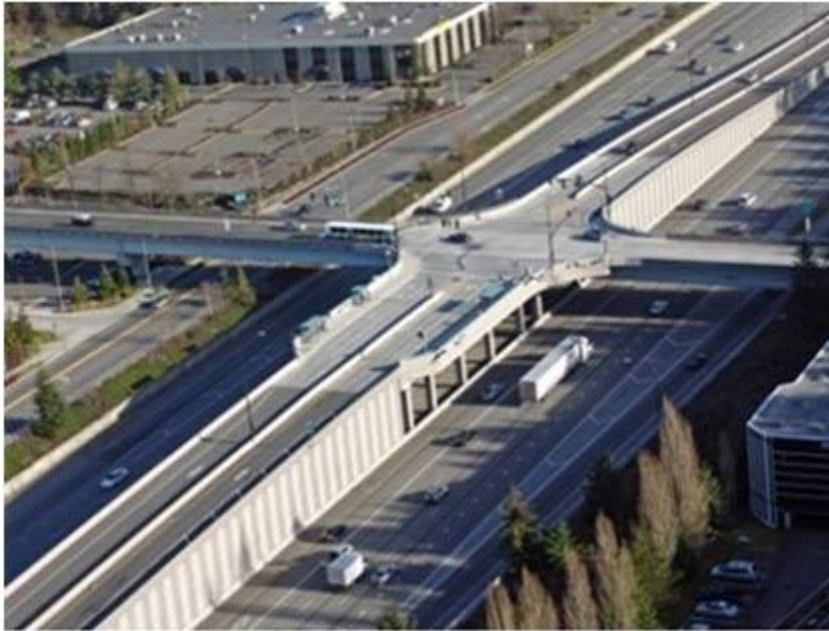
Figure 10: Direct access ramp to HOV lanes in Seattle
