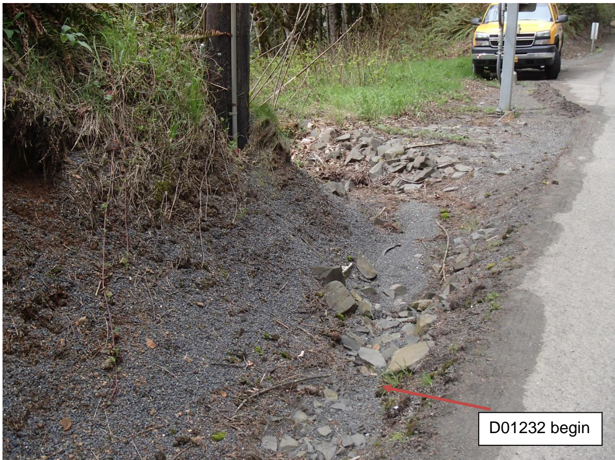
Figure 1: DFI No. D01232, looking west
