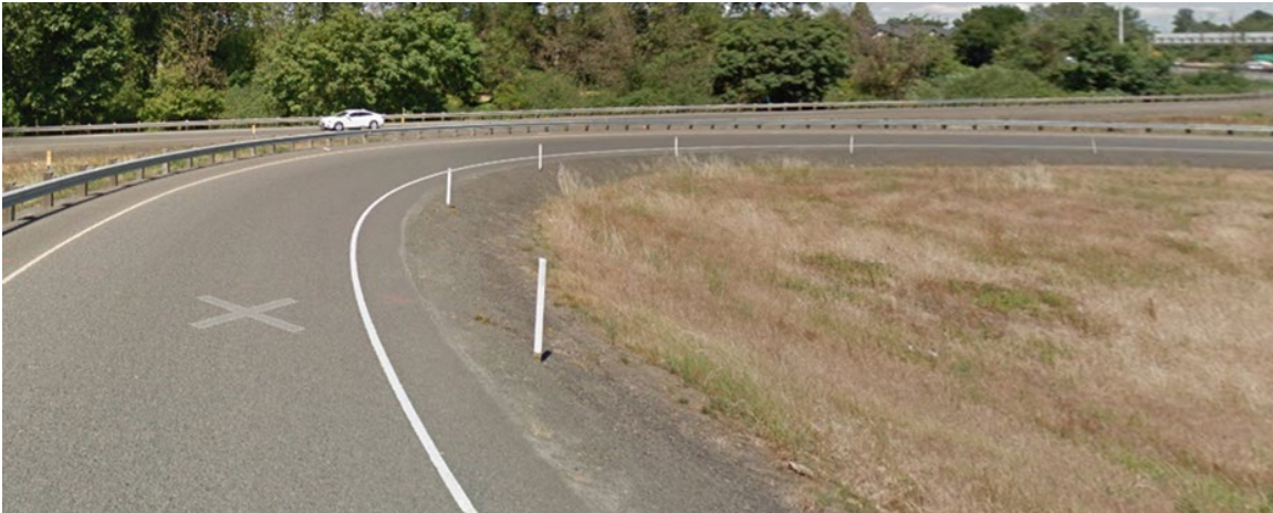
Figure 4: [Placeholder pending facility construction]
