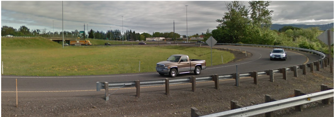
Figure 1: DFI No. D01207, looking North (Placeholder for future photo)
