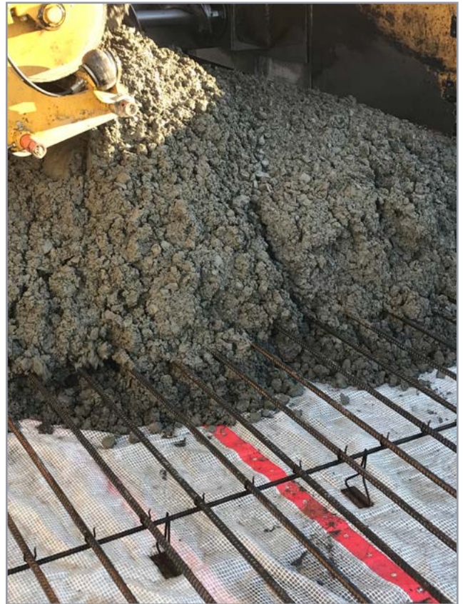
Fig. 6 – Low-carbon concrete installed in I-84 near Meacham.
