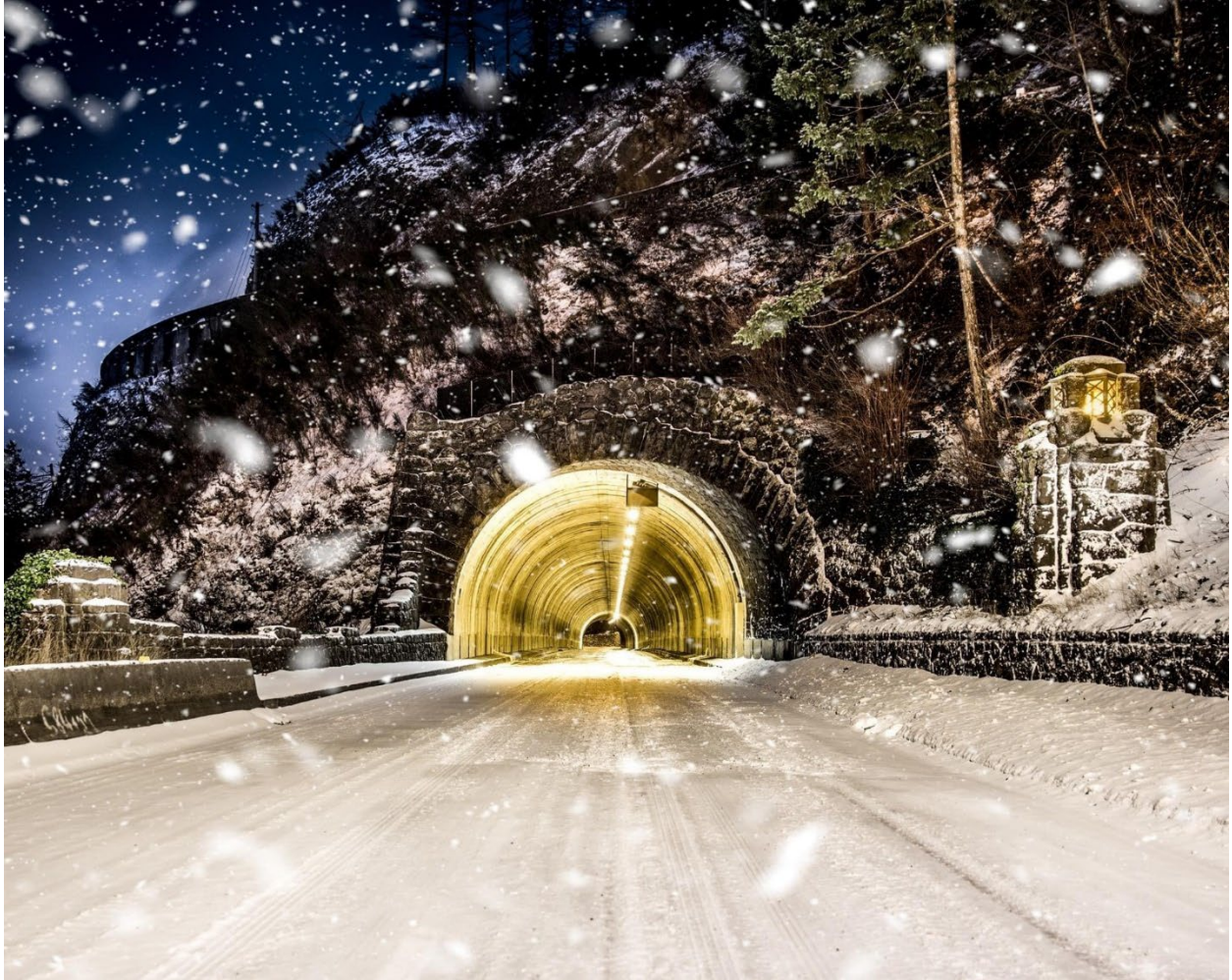
Photo by Jimmy Story , Toothrock Tunnel, Oregon- 2023 ODOT photo of the year
