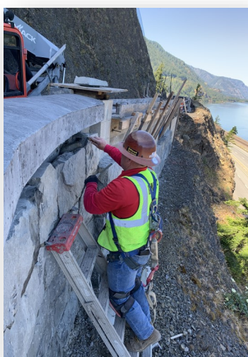
Joint Repair, Concrete Placement in West Portal
