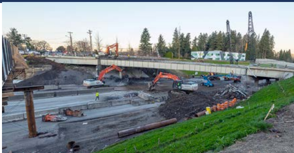
Crews demolish the SW Hall Boulevard overpass in Tigard during a weekend highway closure.
