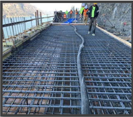
Concrete Placement in Moment Slab At West Bench
