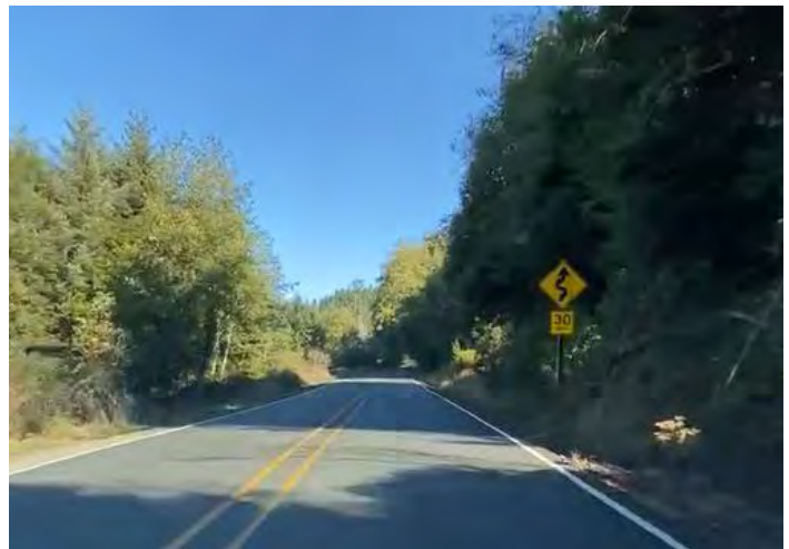
Carpenterville Highway has new curve warning signs to help alert drivers to changes in steep grades and sharp corners. Photo credit: Kittelson
