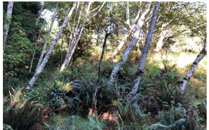
Slumped trees indicate previous ground movement in the central part of the Eighty Acres slide area. Photo credit: Shannon & Wilson
