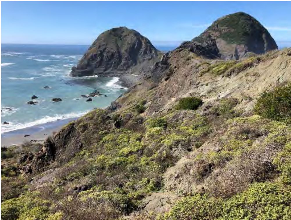
Exhibit 16: Potential recent slope failure along north margin of slide area.
