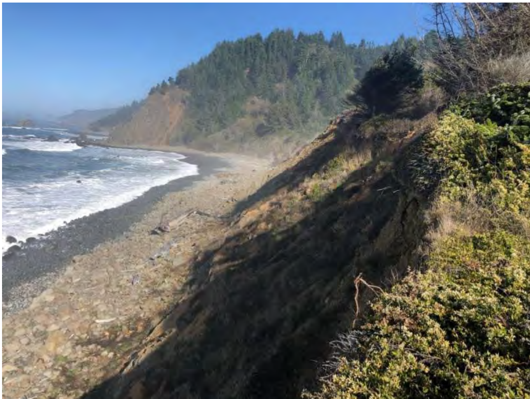
Exhibit 25: Portion of the toe near the coastline being eroded
