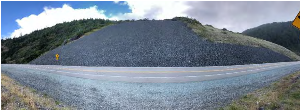
Exhibit 5: Rock buttress along US 101 northbound constructed by ODOT in 2011.
