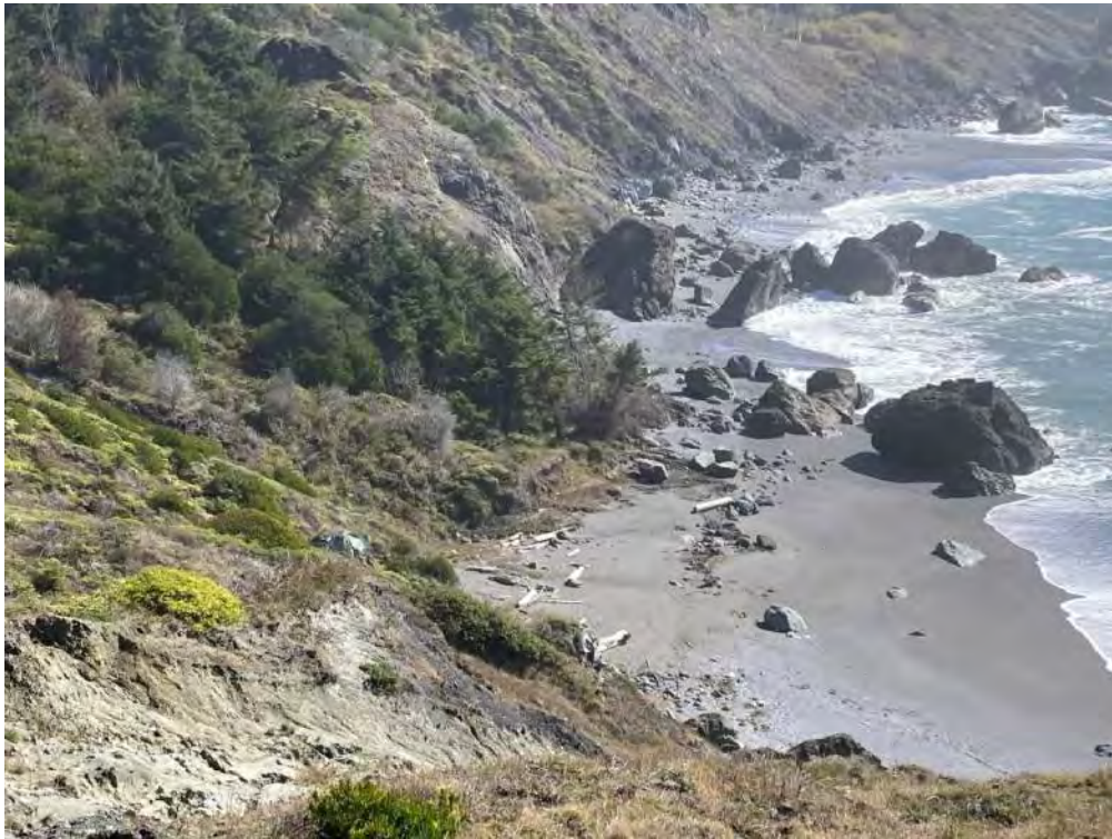
Exhibit 17: Toe of the landslide in the central portion of the photo with slumped trees and disturbed ground.
