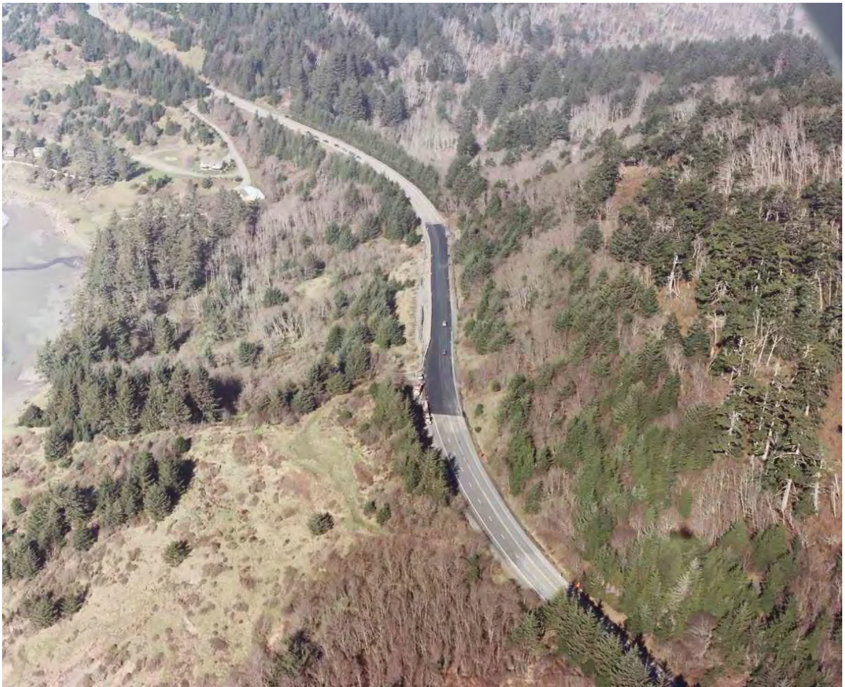
Exhibit 1: Aerial photo looking north at US101 within the Burnt Hill slide limits. The photo shows recent repavement of US101 due to slide activity. Photo taken February 10, 2006.
