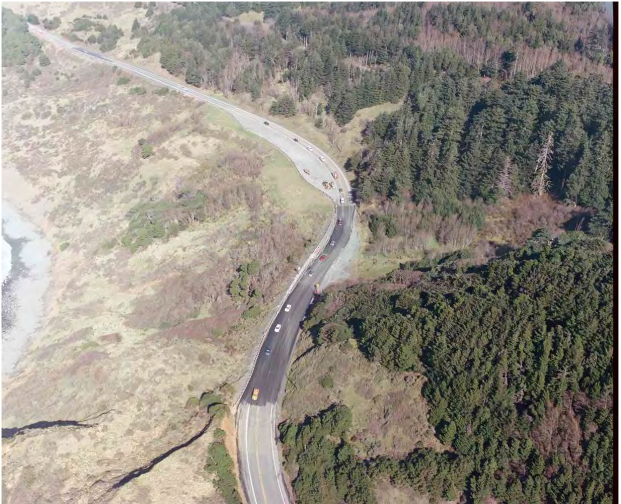
Exhibit 1: Aerial photo looking northeast at US 101 within the Coal Point slide limits. The photo shows recent repavement of US101 due to slide activity. Photo taken February 10, 2006.
