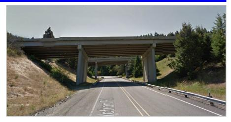
Problem: Constructed in 1965, the I-5 Glendale interchange bridges are in need of seismic strengthening. This project, is part of a larger effort to strengthen bridges and slopes on priority routes to keep southern Oregon connected after a Cascadia Subduction Zone earthquake.
