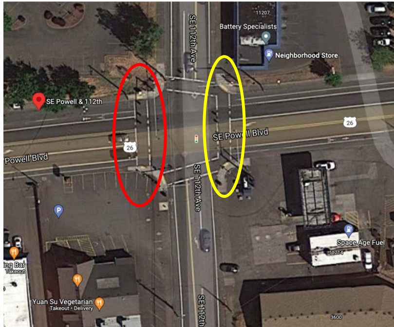
Setback (highlighted in red) and corner (highlighted in yellow) crosswalks at SE Powell Blvd. and SE 112th St
