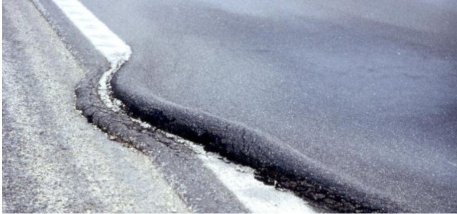
Figure 2.5. Shoving of asphalt pavement due to excessive binder content and low air void in the mix (McDaniel and Levenberg 2013)
