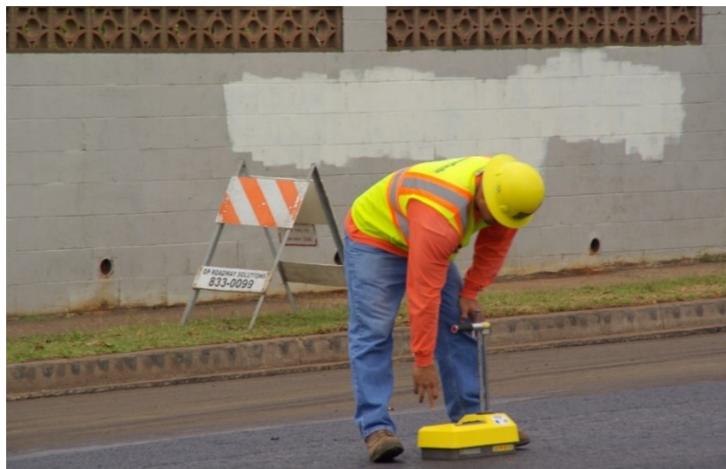
Figure 2.32. Nuclear density gauge in operation (Source: www.pavementinteractive.org )
