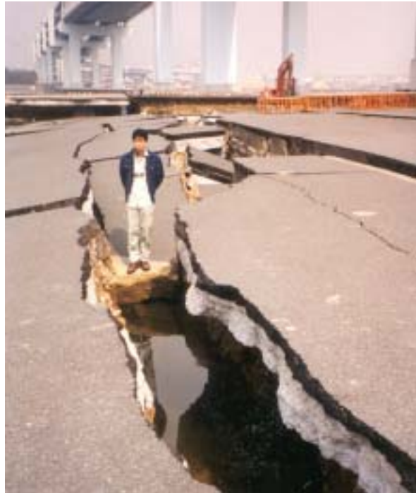
Figure 2.30: Damage to Rokko Ohashi Bridge
