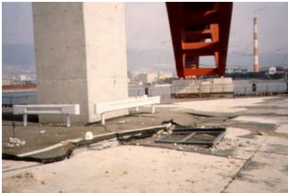
Figure 2.35: Liquefaction Damage Adjacent to the Nadahama Ohashi Bridge
