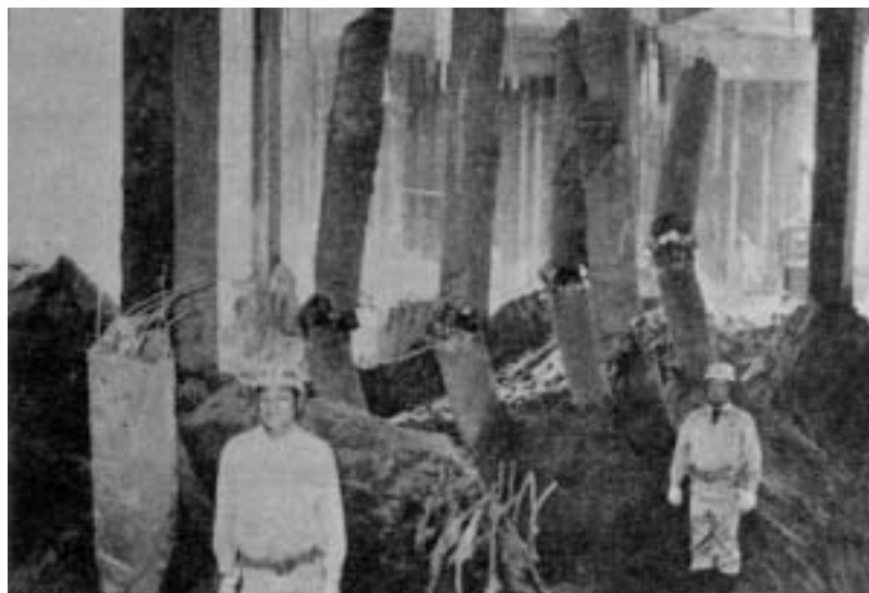
Figure 2.16: Damage to the NHK Building
