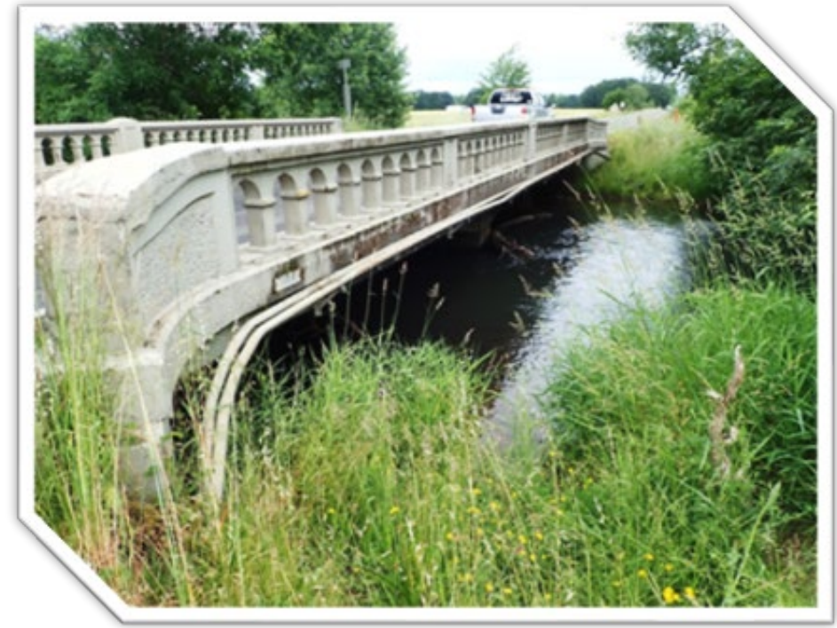
Mill Creek Bridge
