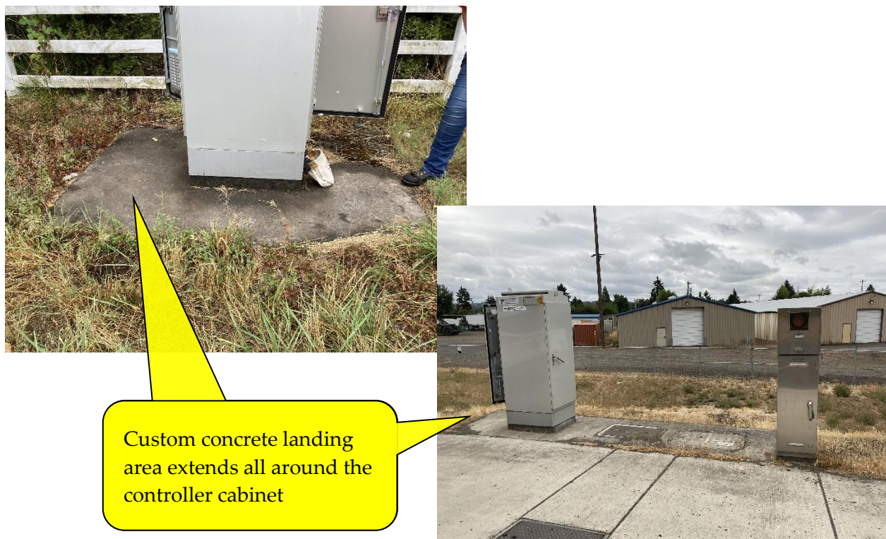
Figure 25-17 | Custom Controller Cabinet Landing Area Examples
