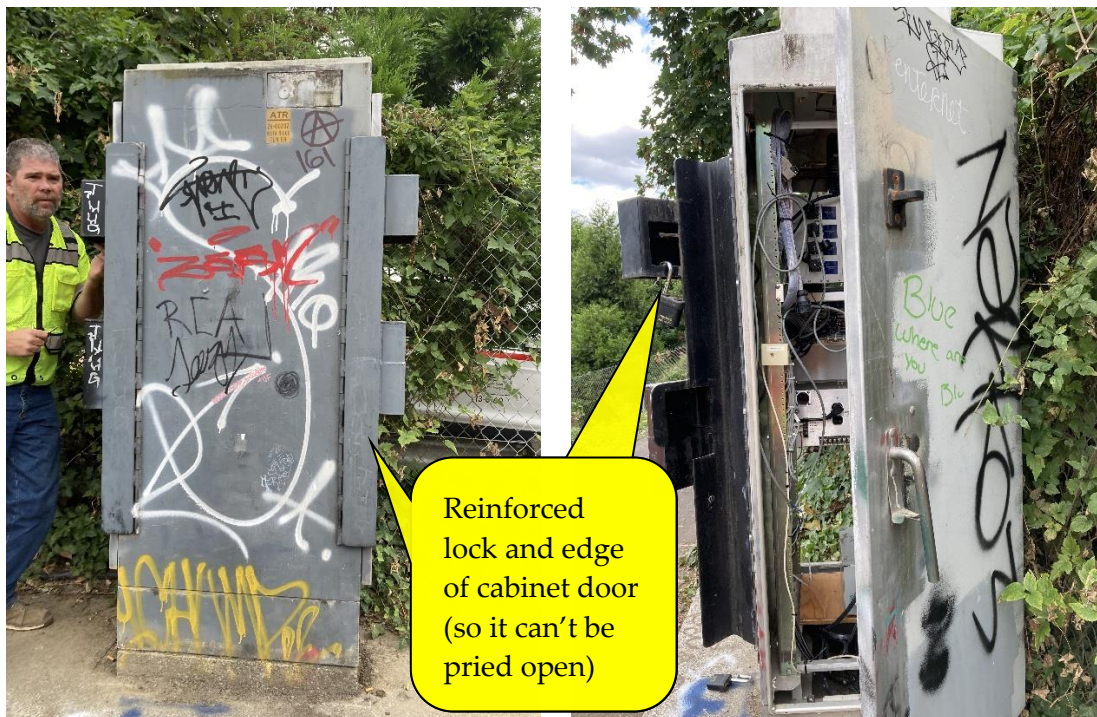
Figure 25-22 | Anti-Vandalism Treatment – Custom Locking Mechanism
