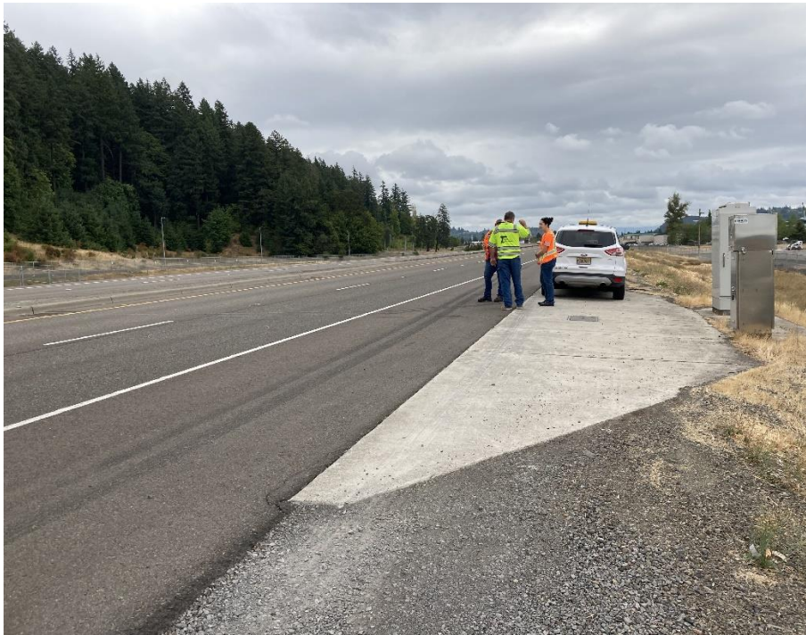
Figure 25-20 | ATR Site Maintenance Pad Example
