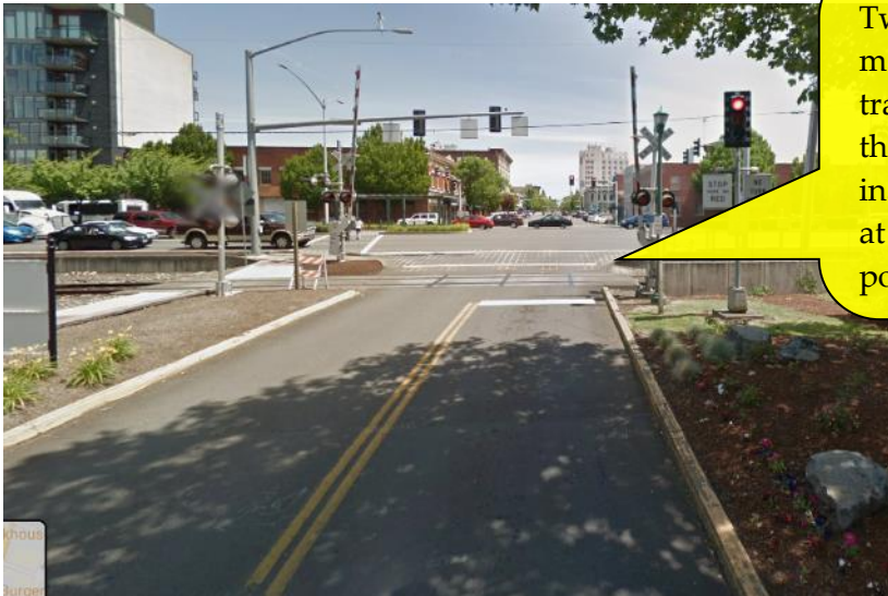
Figure 16-17 | Crosswalk Prior to Railroad Crossing Example 2
