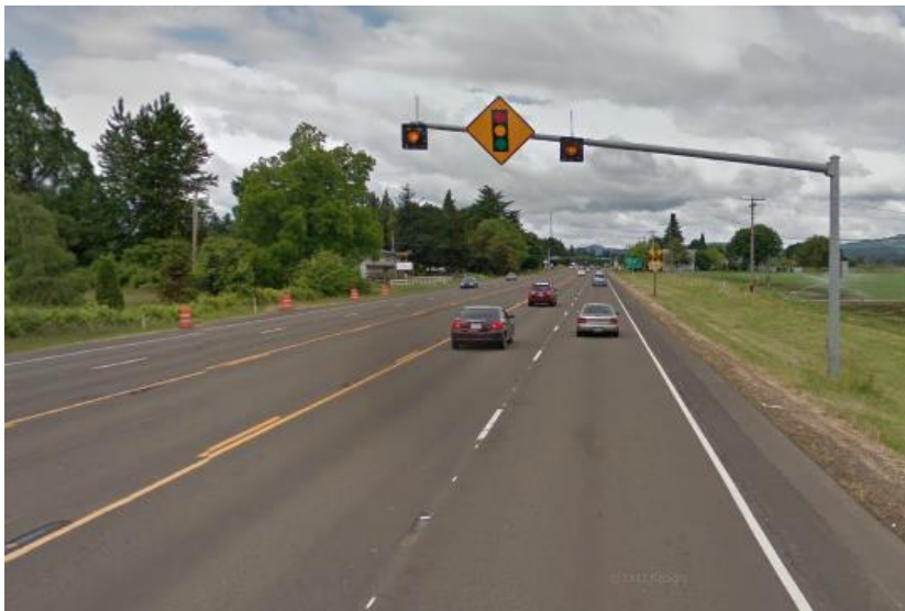
Figure 12-7 | Warning Beacon for a Warning Sign, Overhead
