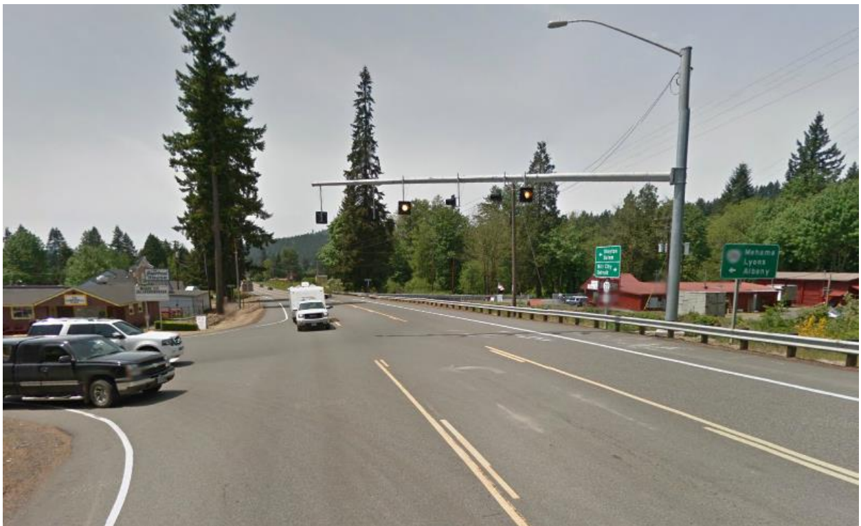
Figure 12-33 | Intersection Control Beacon, Mast Arm, Example 2
