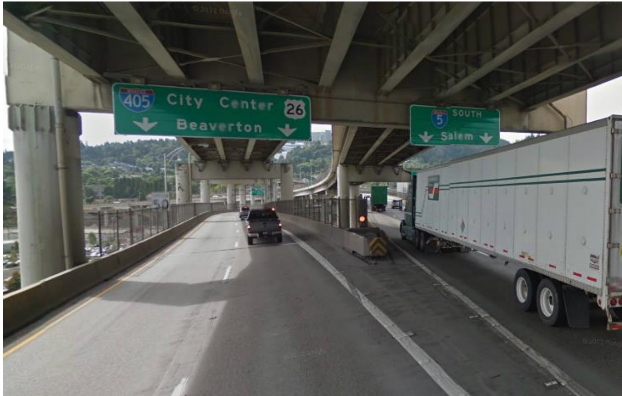
Figure 12-5 | Warning Beacon for an Obstruction, Example 2
