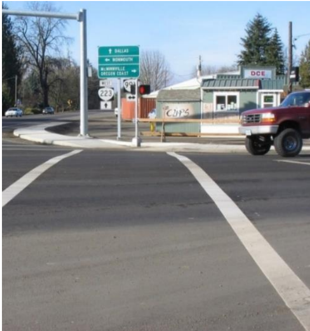
Figure 5-99 | Poor Pedestrian Signal Visibility
