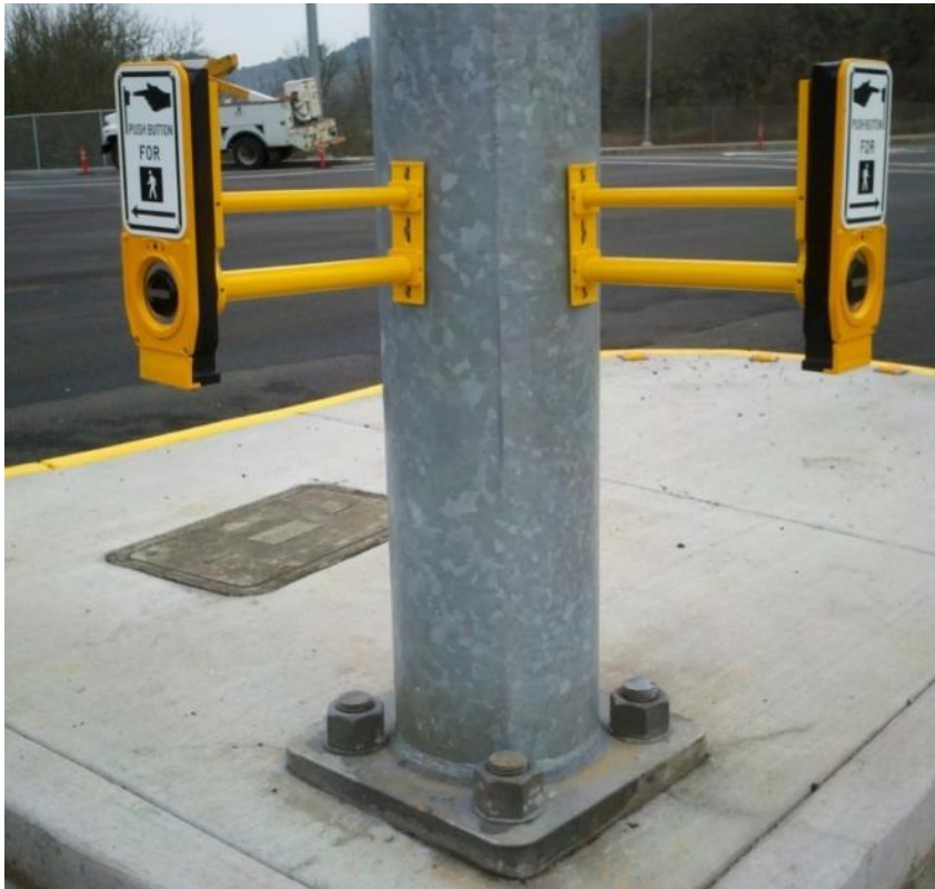
Figure 5-93 | Extension Bracket Mount Example – H-Frame
