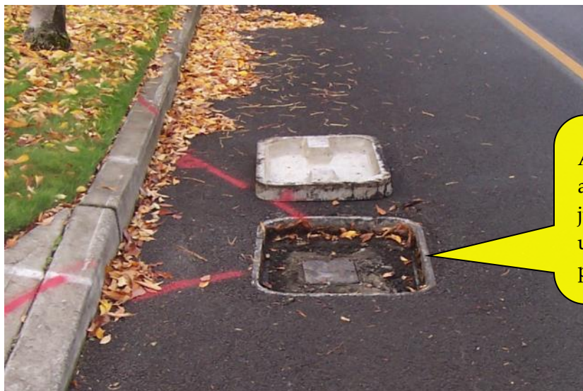
Figure 5-113 | Impacts from Raising Elevation Without Adjusting Junction Box
