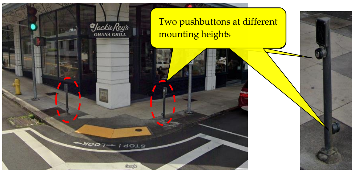
Figure 5-95 | Deviation to Vertical Reach Example
