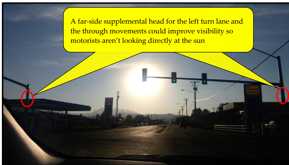
Figure 5-50 | Supplemental Signal Head Placement – Sun Glare Example
