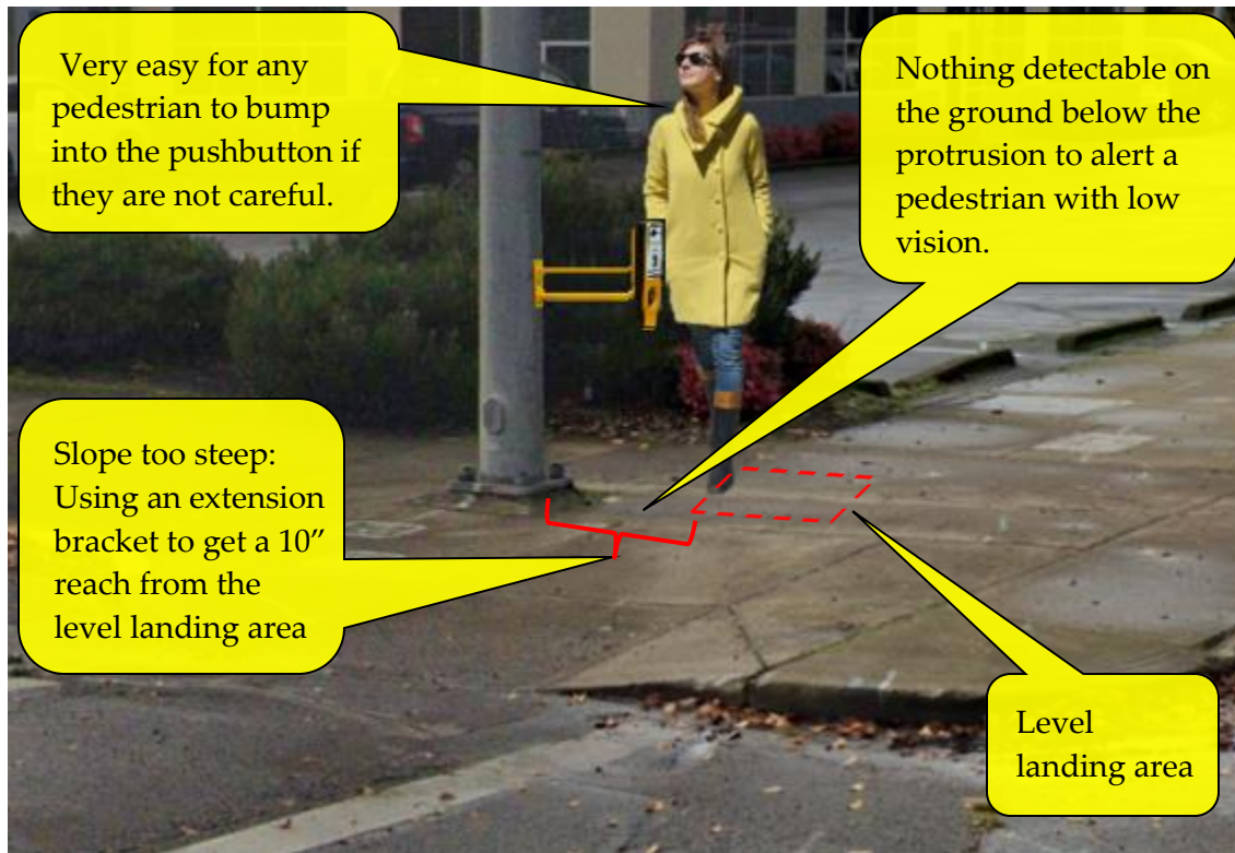
Figure 5-94 | Extension Bracket Mount Photoshop Example – Extending More Than 4 Inches into the Pedestrian Circulation Path
