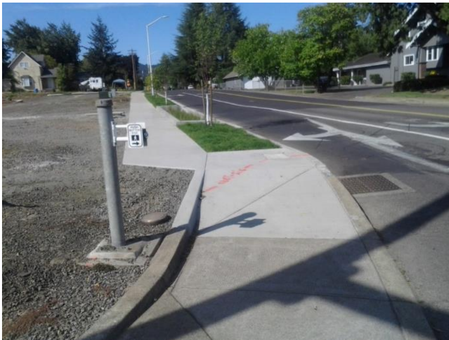
Figure 5-93 | Extension Bracket Mount Example – H-Frame
