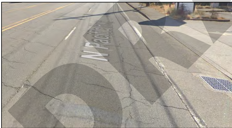
25 26 Figure 5: Edge Line Wear at Minor Driveway (2 of 2)
