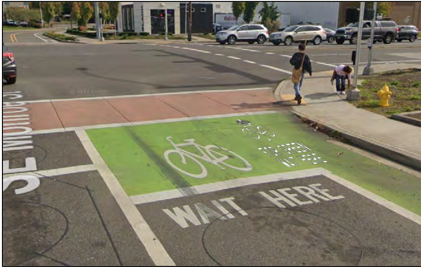
69 70 Figure 3: Proposed Detector Marking at Loop Detector
