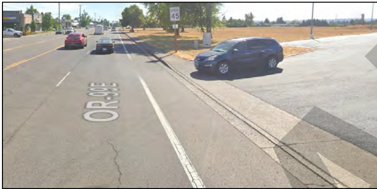
25 26 Figure 5: Edge Line Wear at Minor Driveway (2 of 2)
