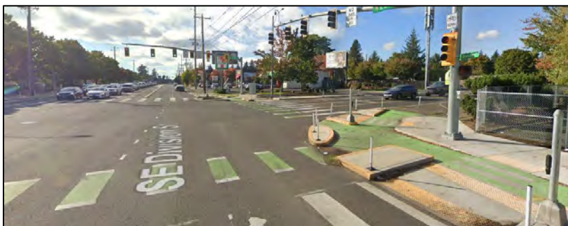
66 67 Figure 8: Bicycle Signal Controlling Separated Bicycle Lanes, Markings and Geometry Showing 68 Allowable Movements
