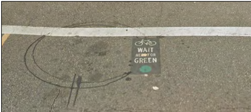
71 72 Figure 4: Proposed Detector Marking in Bicycle Box
