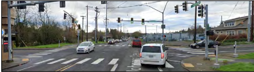
60 61 Figure 6: Bicycle Signal Controlling Painted Bicycle Lane, Markings Showing Allowable 62 Movements
