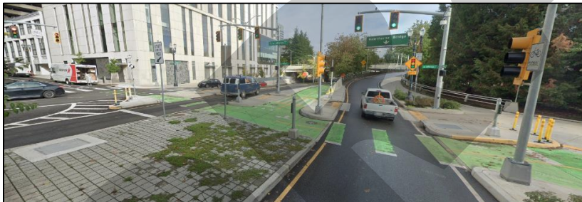
65 66 Figure 8: Bicycle Signal Controlling Separated Bicycle Lanes, Markings and Geometry Showing 67 Allowable Movements
