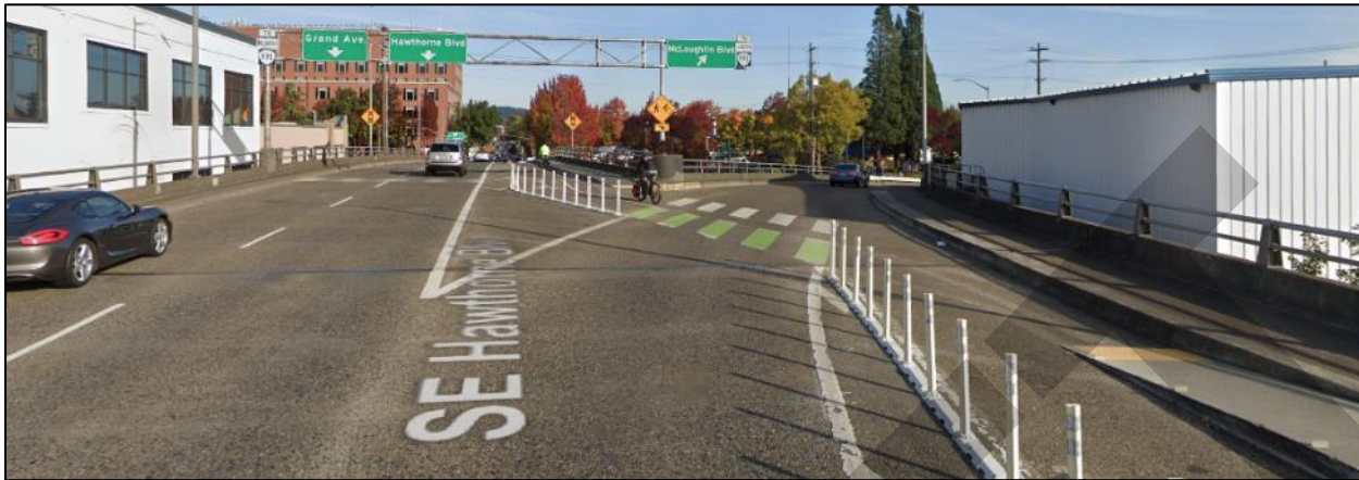
66 Figure 7: Separated Bicycle Lane (curb-separated) to the Right of a Right Turn Lane (right-in-right-out) 67
