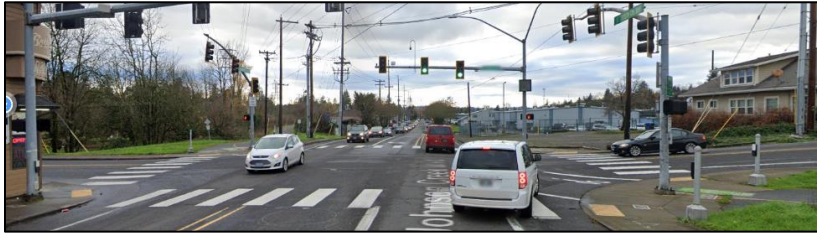
59 60 Figure 6: Bicycle Signal Controlling Painted Bicycle Lane, Markings Showing Allowable 61 Movements
