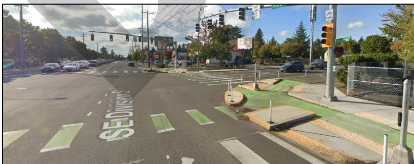
65 66 Figure 8: Bicycle Signal Controlling Separated Bicycle Lanes, Markings and Geometry Showing 67 Allowable Movements
