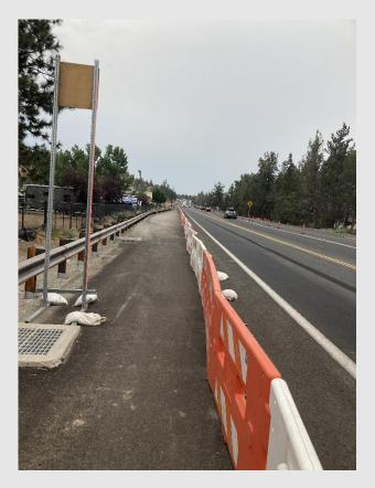
Provide non-slip, 60 Inch minimum wide surface through entire pedestrian route. If not possible, provide 48" min. width with 60" x 60" passing spaces every 200 feet along the route.
