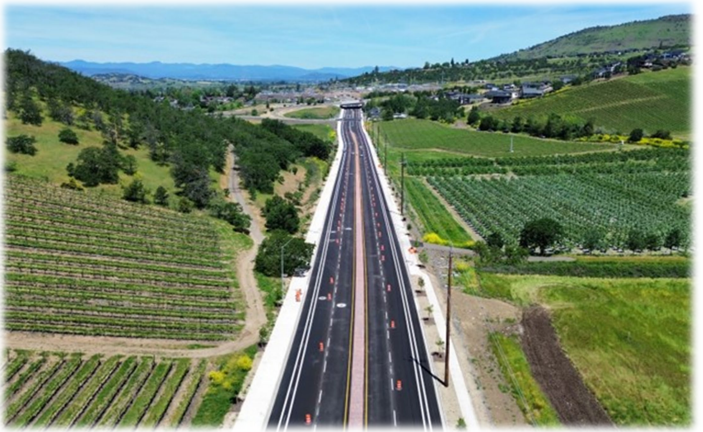
City of Medford, Foothill Road Project
