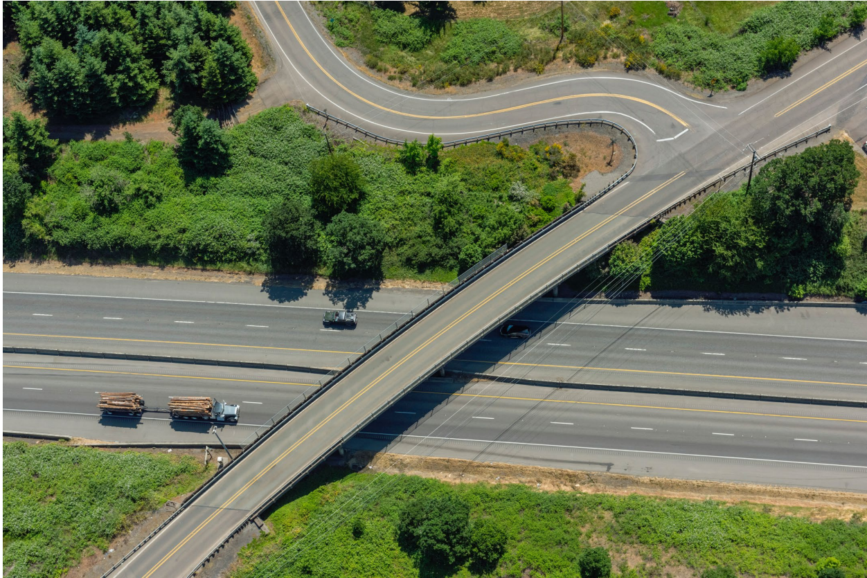
Figure 4 Existing Battle Creek Rd Overcrossing without bike/ped facilities or shoulders.
