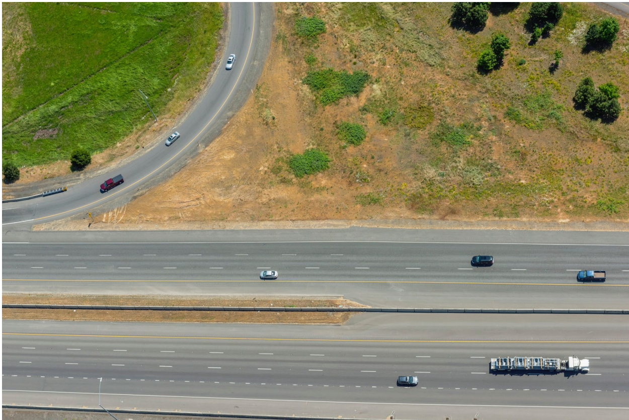
Figure 3 I-5 NB Transitions from two lanes back to three at Kuebler Blvd Interchange.
