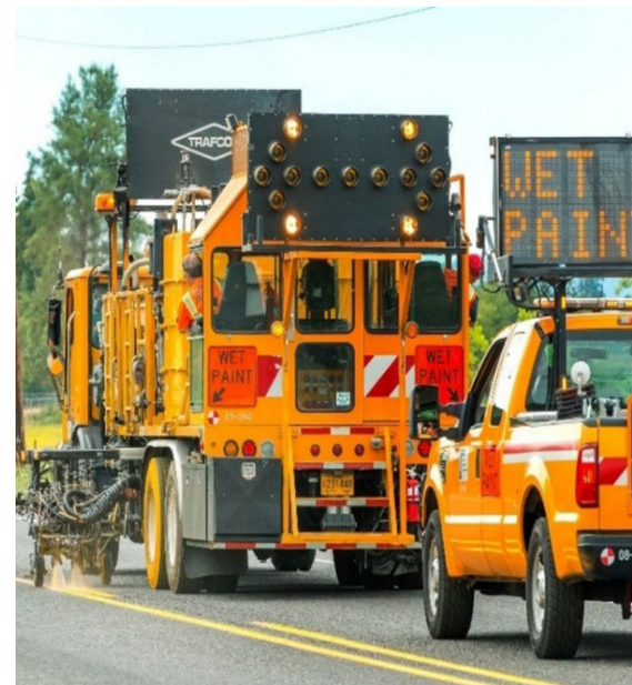
Maintenance work helps us identify and mitigate small issues before they become big problems.
